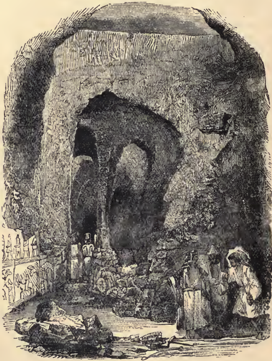
Underground Excavations at Kouyunjik.
